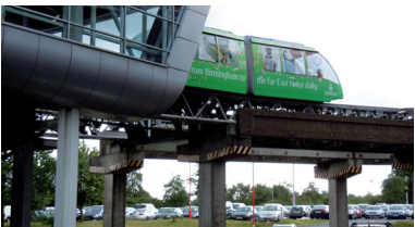
Elevated steel guideway utilizing the pre-existing concrete structure.
